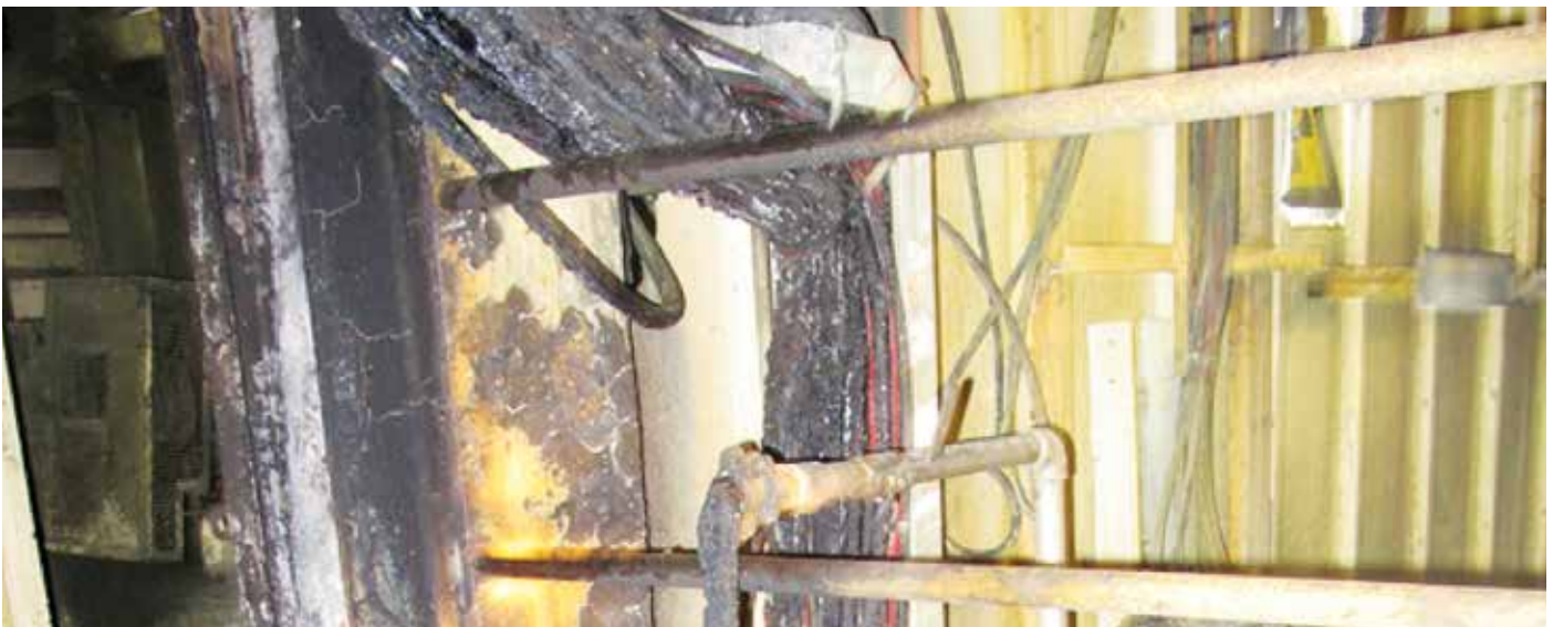
Electrical wiring was destroyed inside the Final Recovery Plant during the February fire.
