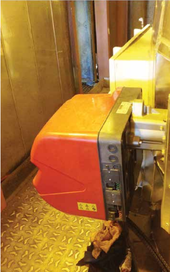
New burner installations.
