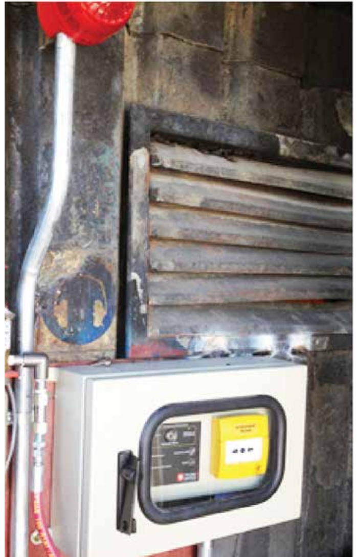
New manual activation suppression system.
