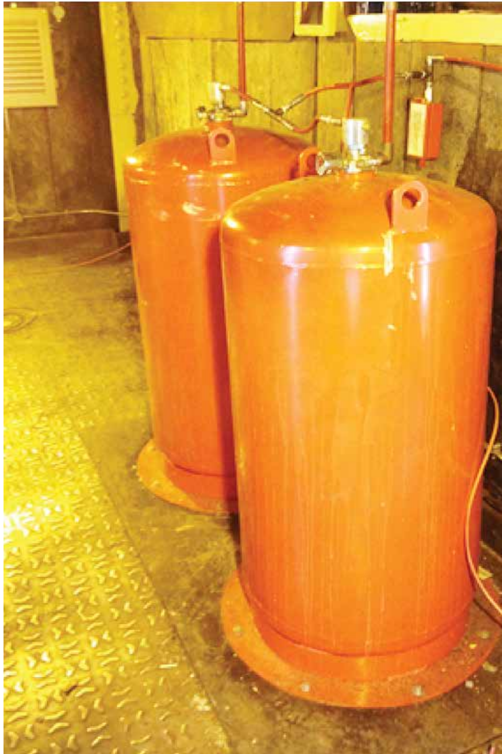
New Final Recovery Plant fire suppression system.
